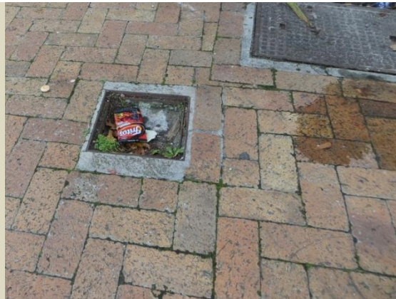
Figure 19 Broken manhole covers on sidewalks
