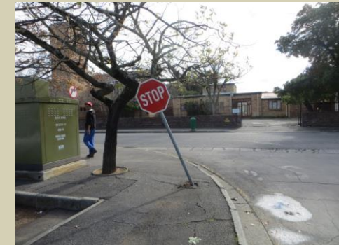
Figure 16 Bent and disorientated signage
